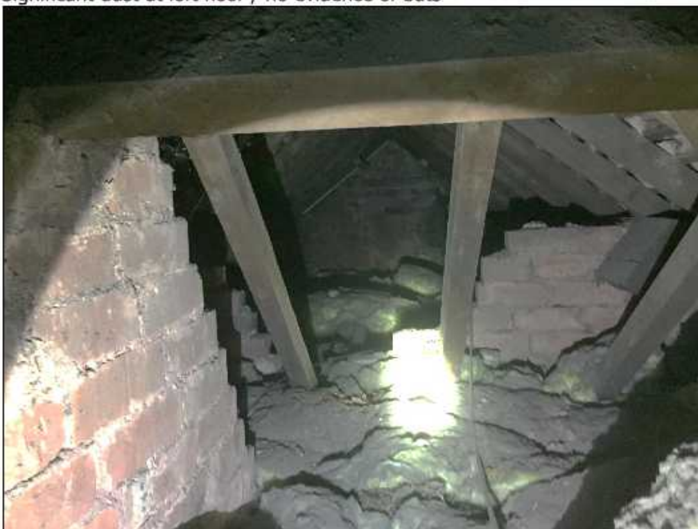
Significant dust at loft floor / no evidence of bats
