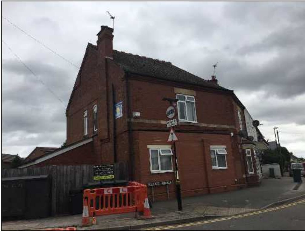
Western elevation well-sealed roof
