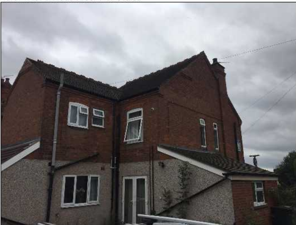
North elevation well-sealed roof
