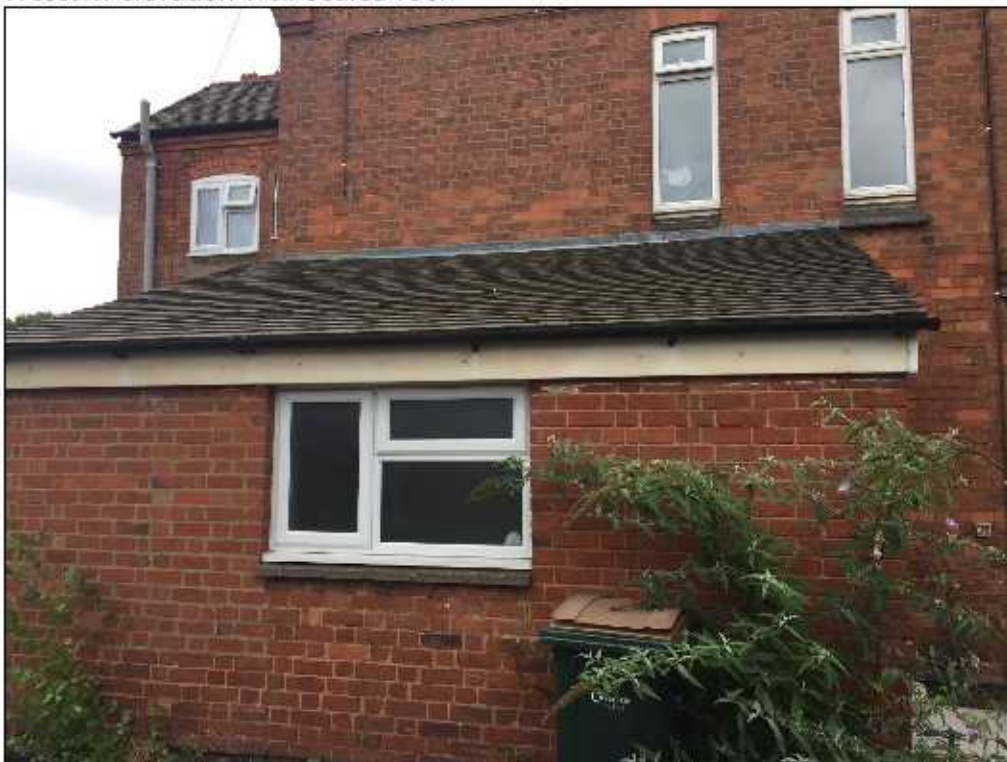
Lean to well-sealed
