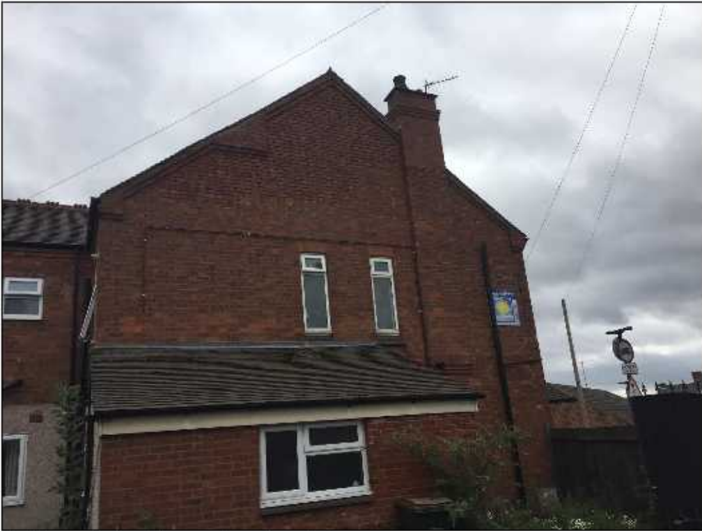
North west elevation roof well-sealed
