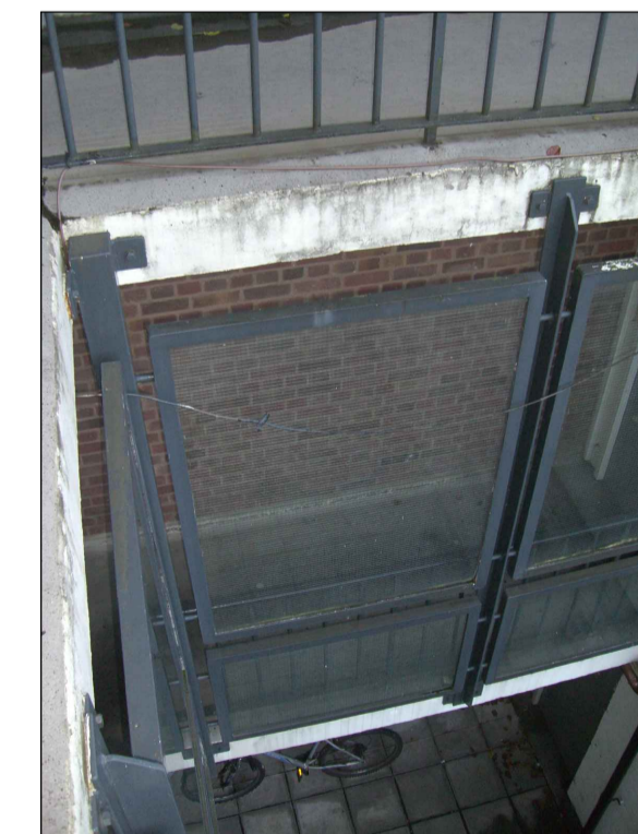
C. Existing screen at lower level
