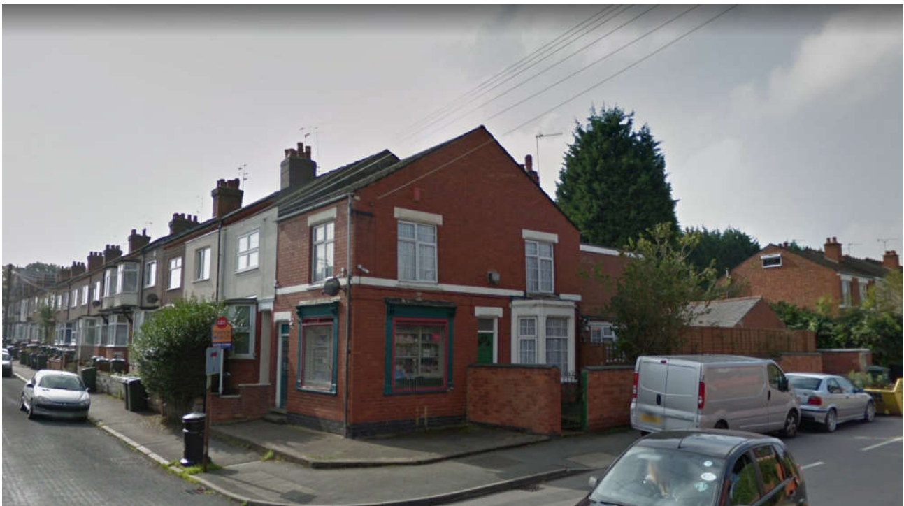
Figure One: view of the corner property, 60 Kingsland Avenue.
